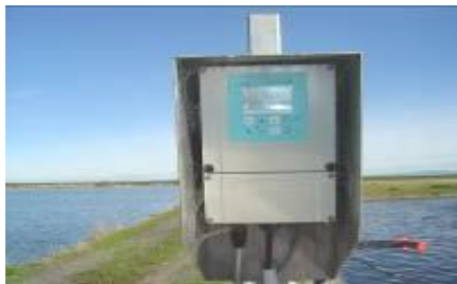
Image: Aeration Pond DO meter
