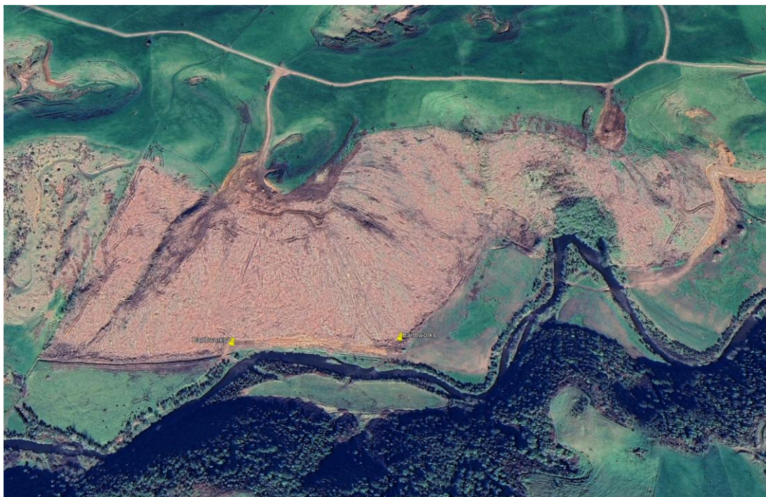
Figure 1.1. Tree felling and earthworks on the Mangatutu Stream January 2024.
