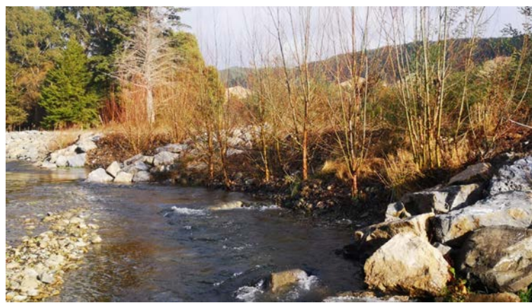
^ Improving channel diversity within the lower Motupiko through use of alternative approaches to riprap – in this case rock groynes interplanted with matsudana willow poles from TDC's nursery. Photo: Rhys Barrier
