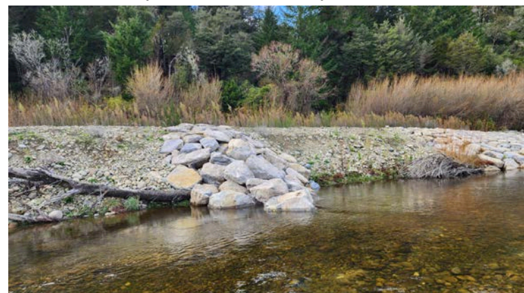
^ Recently constructed spur groynes with layered willow near water line to assist with summer thermal mitigation of rockwork through both shading and improving instream channel diversity. Photo: Jacob Lucas
