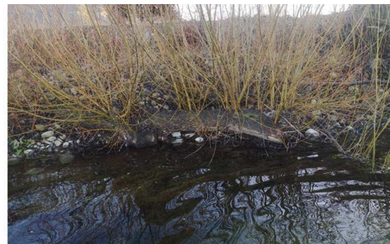
^ Excellent use of buried in-situ willow material during past erosion repair works – a live willow bank at waterline now exists to stabilise bank area between rock groynes and provide overhead shading for the pool habitat created by rock groyne placement. In addition, fish cover and a terrestrial insect source for aquatic life has also been created. Photo: Rhys barrier
