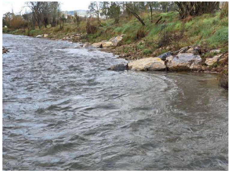
^ Groynes in the Dove River, seen during a winter spawning survey. Photo: Rhys Barrier.
