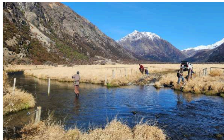
^ Rainbow side-stream fence repairs. Photo: Jacob Lucas
