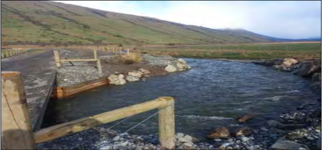
Photo 1. Showing the Glenariffe South Branch being re-directed into the East Branch, and restoring an unbroken Glenariffe Stream.
