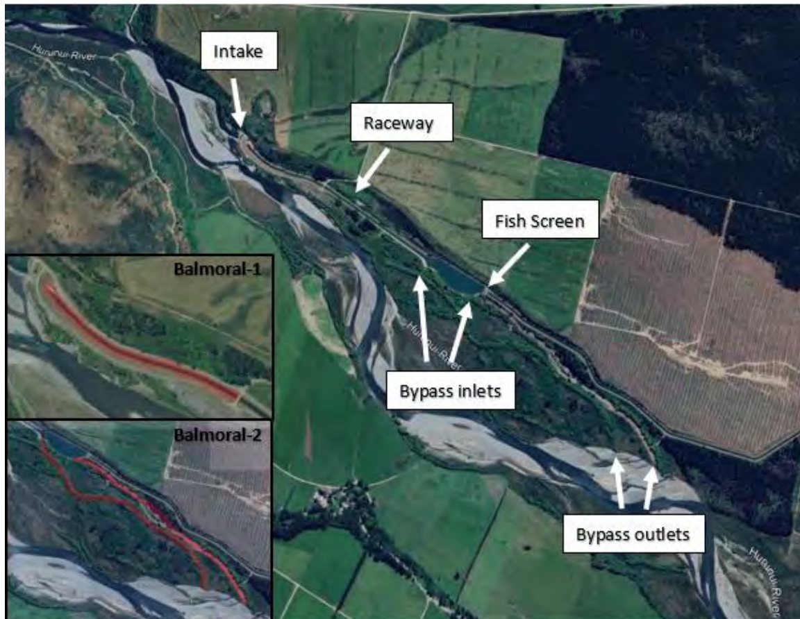
Figure 3. The Balmoral scheme on the Hurunui River. Insets show the upper and lower (bypass) focal sections highlighted in red.
