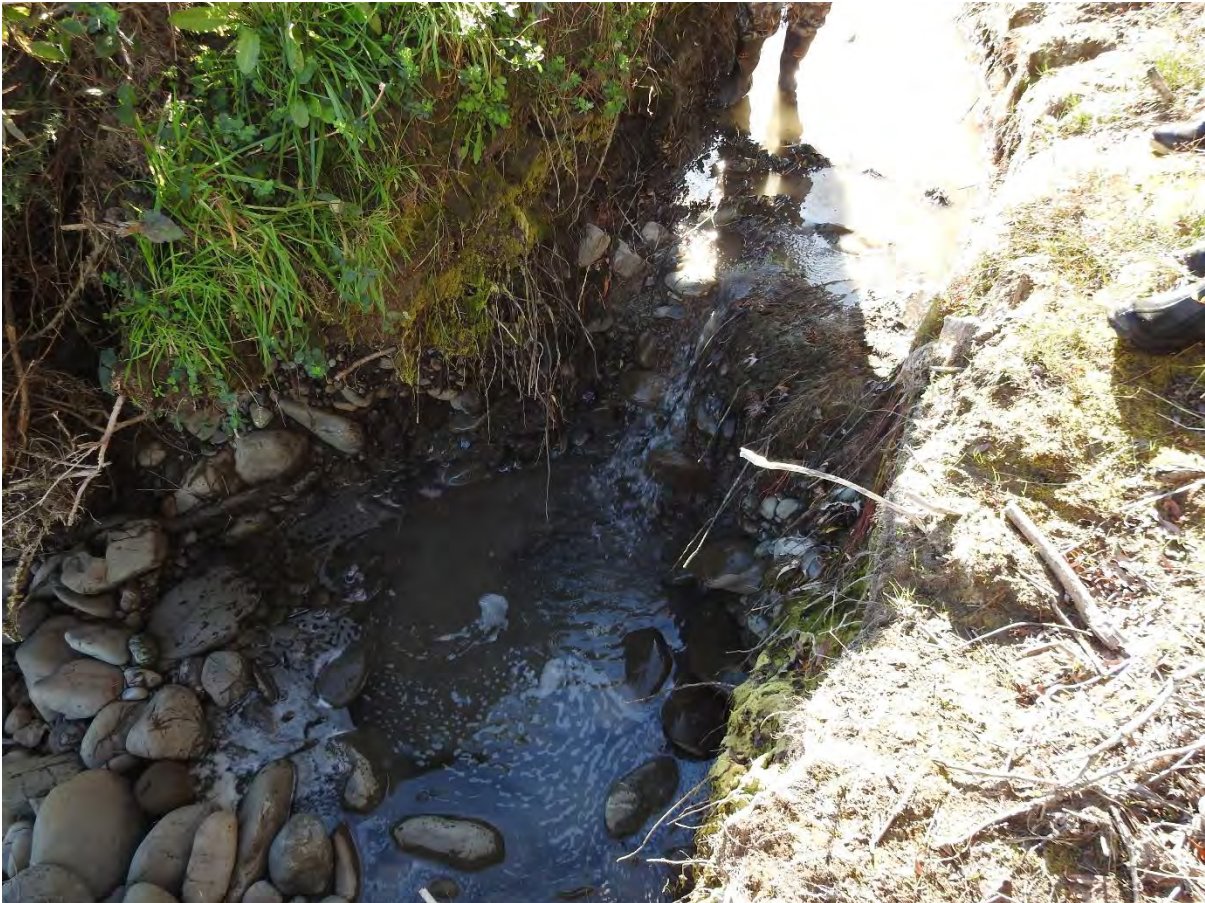
Figure 6. Outlet of lower bypass channel of Balmoral irrigation scheme where it meets the Hurunui River riverbed .
