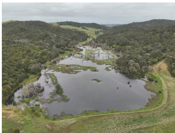
Stage 2 of Underwood Wetland development taken from drone
