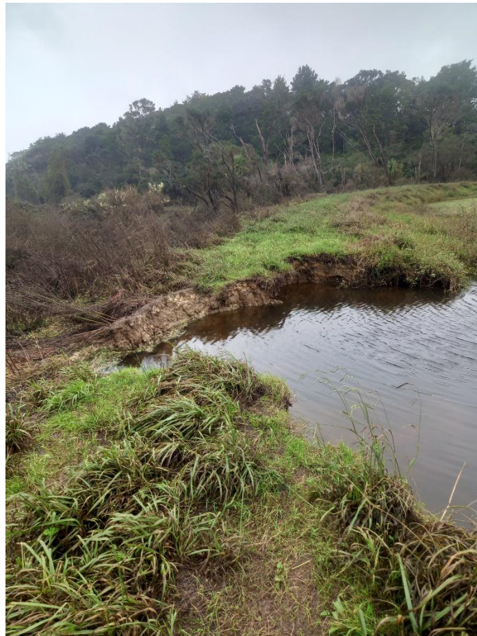
The bund breach in the big pond at Jack Bisset Wetland
