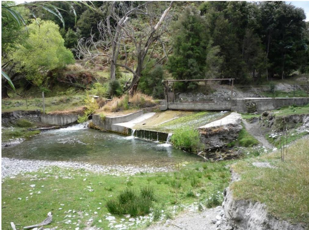
*Figure 2: Showing the concrete dam structure and Guillotine
