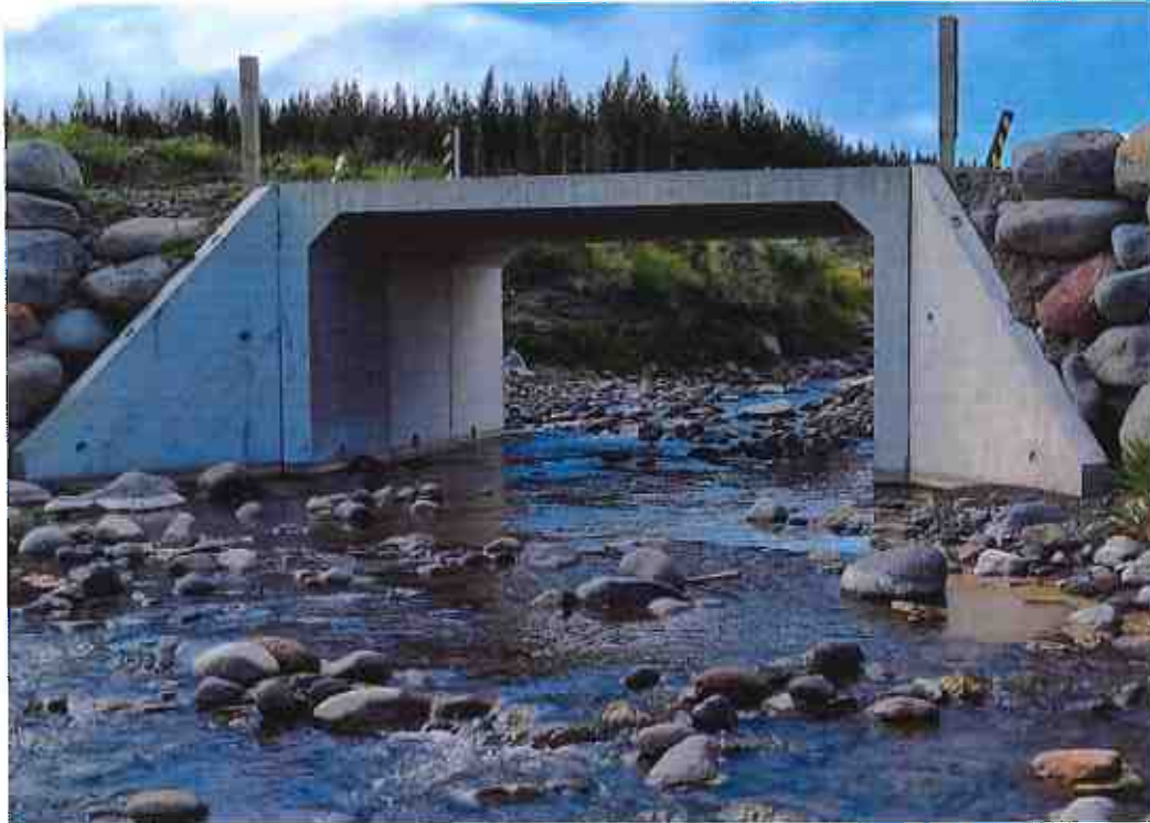
Photo 15: Tokiahuru Stream tributary Link Road box culvert (Site 8), 5 th December 2024.
