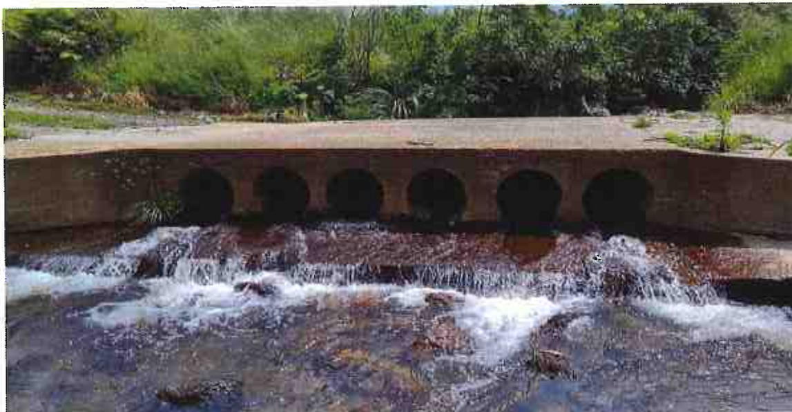
Photo 26. A six-barrel concrete ford in Mangatengehu Stream at Derby Road (Site 5).
