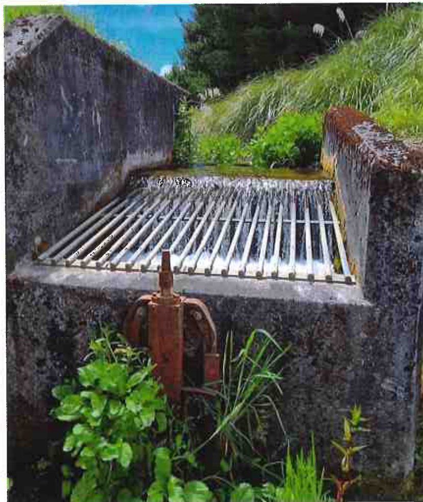
Photo 11. Wāhianoa River tributary - Aqueduct Road intake, 4 December 2024.
