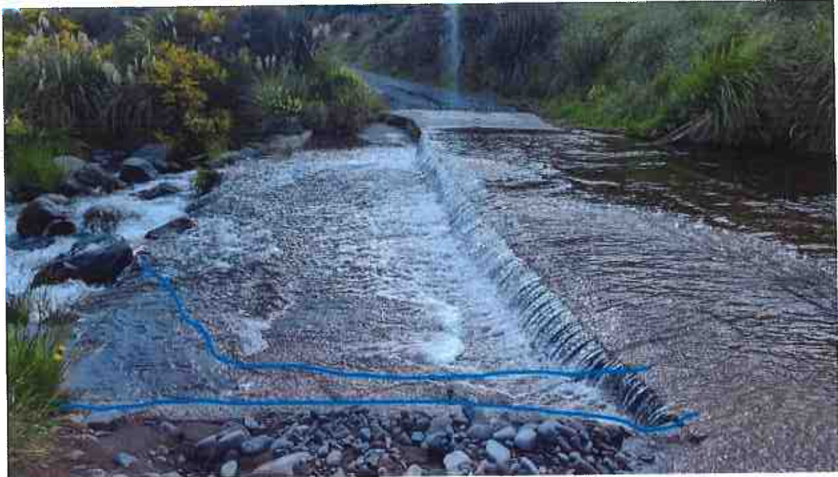
Photo 14. Potential fish passage pathway (in blue) that could be enhanced to provide for upstream fish passage at low flow.
