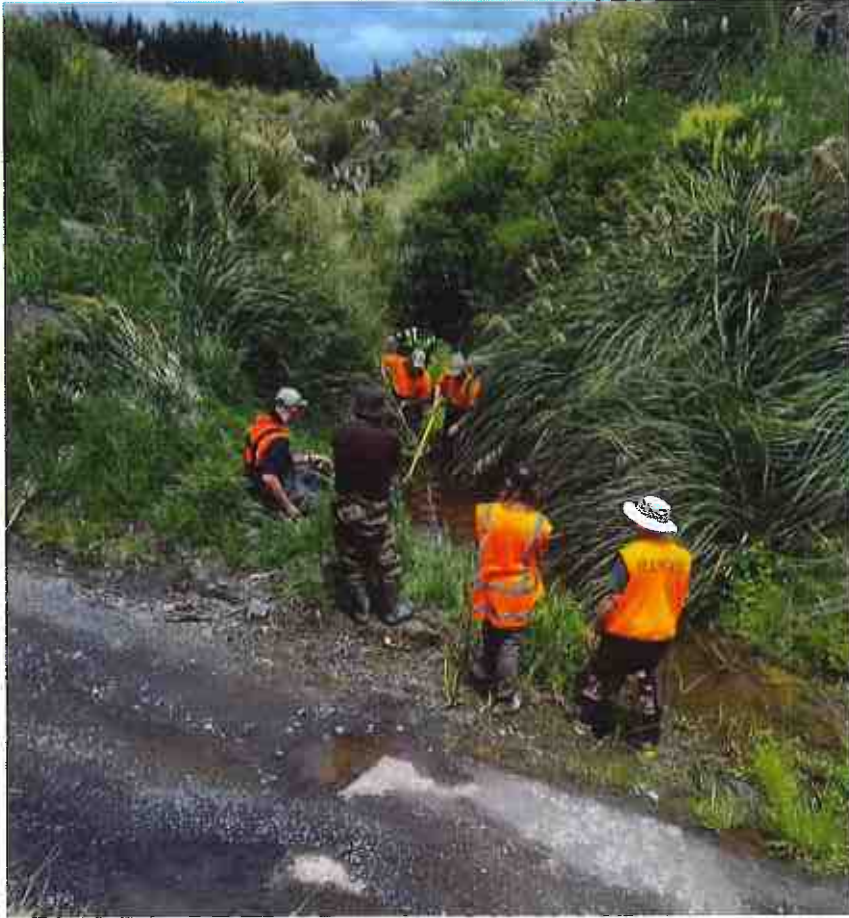
Photo 12. Wāhianoa River tributary - Aqueduct Road intake, fishing the downstream seepage flow, 4 December 2024.
