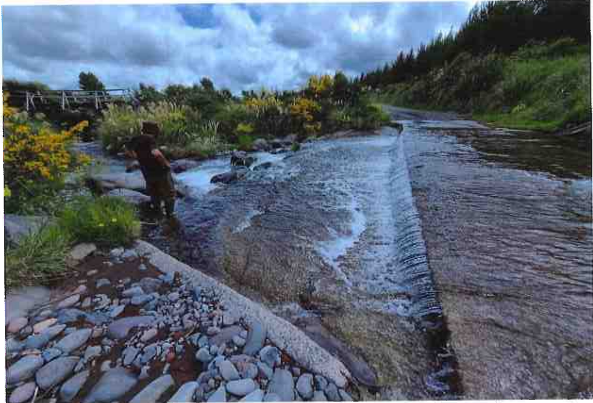
Photo 9. Wāhianoa River W 1 Lower Ford crossing (Site 3) looking downstream, 4 December 2024.
