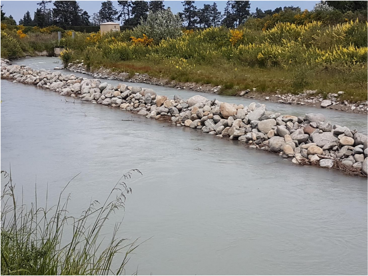
Rock Bund Fish Screen – Irrigation industry now agree these are ineffective and difficult/expensive to monitor
